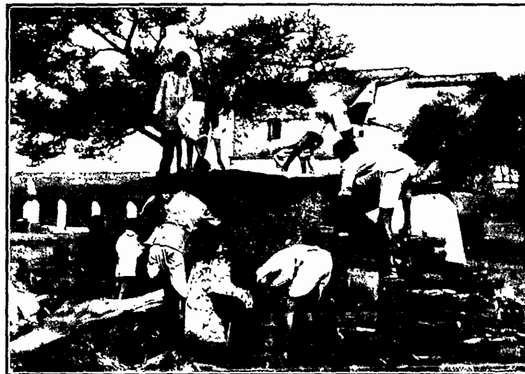
Boys of the Methodist school at Vikarabad, Deccan, preparing a kiln of lime for burning.
