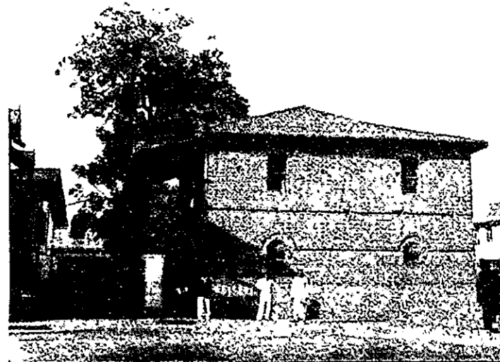
The rented house referred to in this booklet as the makeshift for a Parsonage and Chapel, in the city of Ahmedabad, India. The half of the upper storey to your right is the Chapel room. But only 60 or 70 of the 500 Christian mill-hands can get in.
