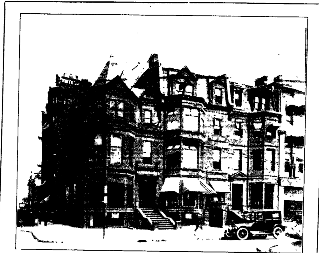
DEPARTMENT OF RELIGIOUS EDUCATION AND SOCIAL SERVICE OF BOSTON UNIVERSITY, ON COPLEY SQUARE, BOSTON Latest Development in Educational Work, Devoted to Training Men and Women for Service in City, in Rural Sections, and Among the Non-English
