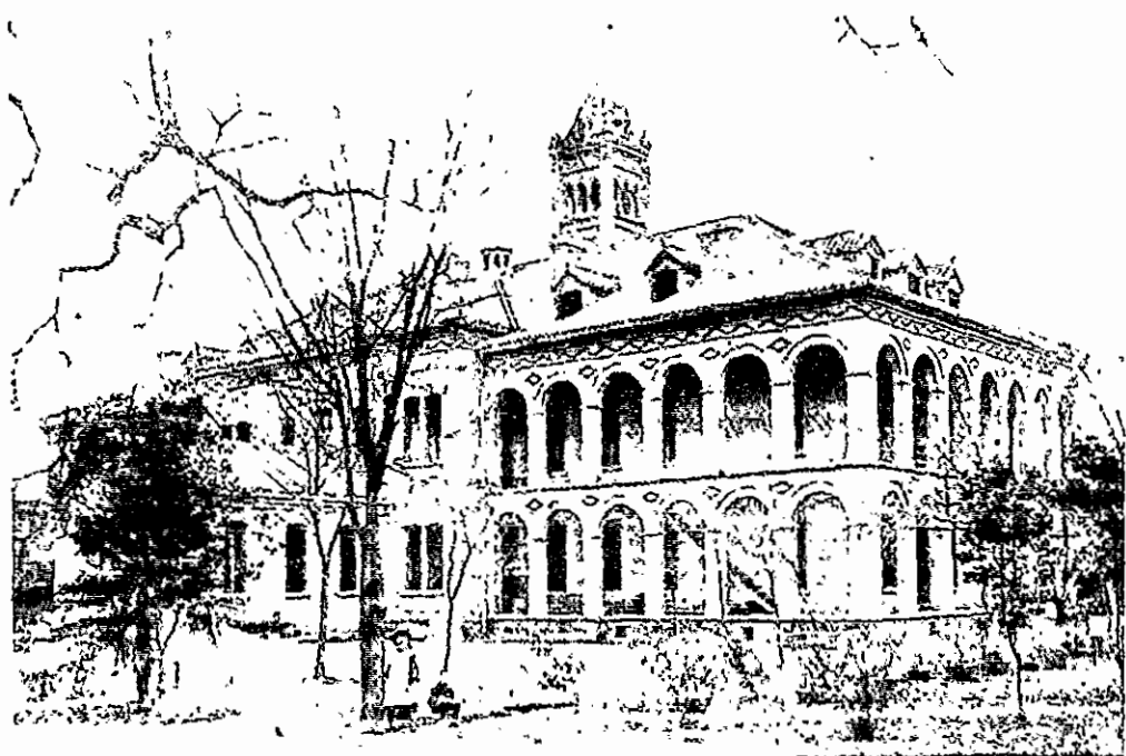
THE HOSPITAL AT CHENTU, WEST CHINA
